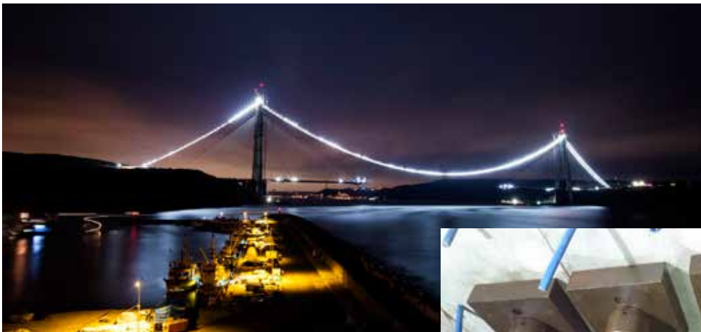
Yavuz Sultan Selim Bridge (aka Third Bosphorus Bridge) Designer Hyundai & SK Engineering JV Installation and Stressing by Intekno
