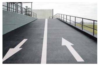
Ramps and entrances are some of the areas in a multi-storey car park which are most subject to high mechanical loads. However, if the car park is being refurbished, these areas cannot be closed for extended periods without considerable disturbance. Triflex systems cure quickly and can be opened up to traffic
