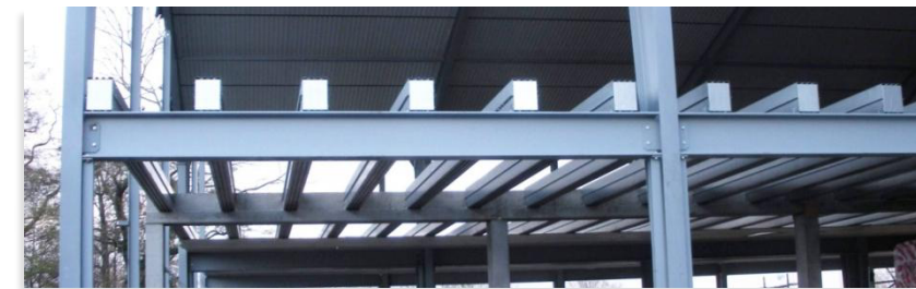
Roof elements and floor beams.
