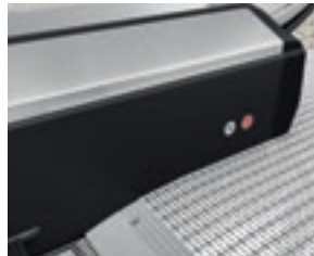
Sheet steel skirt with black anti-friction coating
