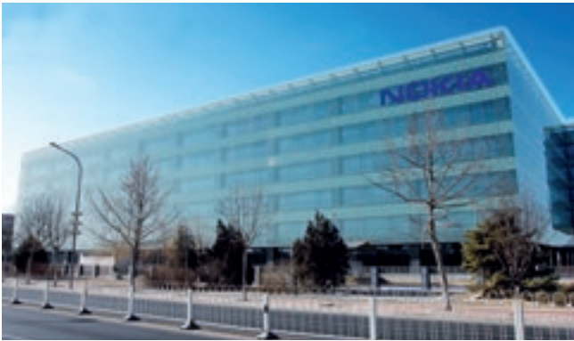
Nokia Headquarters Business Building, Beijing, China
