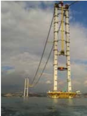
Yavuz Sultan Selim Bridge (aka Third Bosphorus Bridge) Designer Hyundai & SK Engineering JV Installation and Stressing by Intekno
