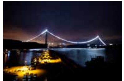
Izmit Bay Bridge Main Contractor IHI
