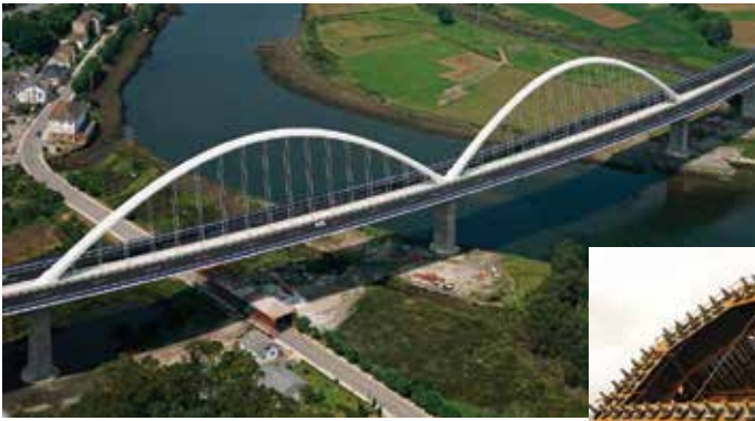
Navia River Viaduct, Spain Post Tensioning Sub-Contractor BBR PTE
