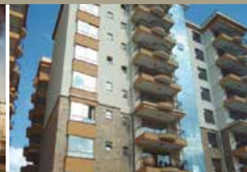
Skyview Towers. KENYA
