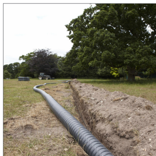
RAUVITHERM installation
