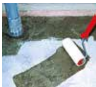
1. Prime wall junction and surface.
