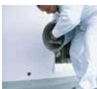
5. Spread the surface coating Triflex ProFloor ...
