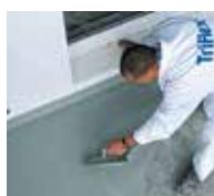
6. ... using a trowel, and ...
