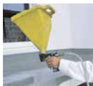
10. ... blow in Triflex Micro Chips.
