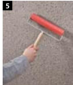
5 Press the sand mixture into the soft plaster using the Sto-Terrazzo Effect Roller. In areas that are difficult to reach, use a square trowel.
