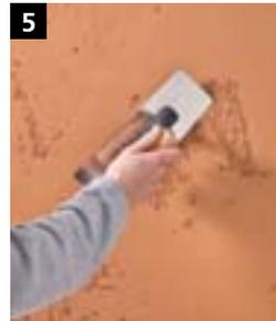
5 Carefully smooth the surface using the edge of the StoCalce Marmorino Smoothing Trowel. Leave the surface to dry until it is touch-dry.
