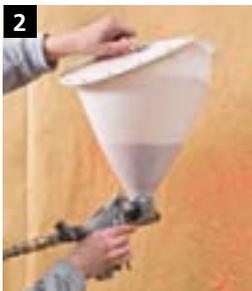
**2** Dilute StoLook Texture G (colour shade 14DC180) to 7 % with water. Pour the material into the Sto-Hopper Gun (6 mm nozzle). Set the air pressure to 0.5 - 0.8 bar and determine the amount of material on the hopper gun. Define the spray pattern on a test surface.
