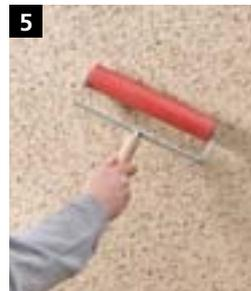
5 Press the sand mixture into the soft plaster using the Sto-Terrazzo Effect Roller. In areas that are difficult to reach, use a square trowel. Leave to dry.
