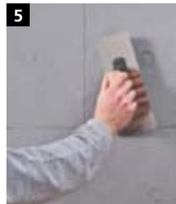
5 Leave the surface to dry slightly and compact using the edge of the StoCalce Marmorino Smoothing Trowel. Leave to dry.
