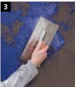
3 Apply large spots of StoDecolit MP (colour shade 14DC120). Decant the material on the surface and smooth into one spot using a Sto-Smoothing Trowel held flat. Layer thickness of the spotted coating approx. 1 - 1.5 mm.
