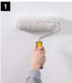
**1** Apply two coats of StoColor Opticryl Gloss (colour shade white) over the full surface using a short-pile roller. Leave to dry.
