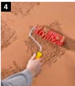
4 Immediately create a partial texture with the Sto-Relief Roller "Oak" on the surface to suggest the shrinkage holes. Leave the surface to dry briefly.
