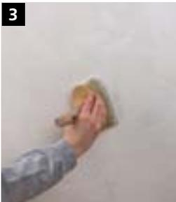
**3** Working in cross-wise motions again, apply a mixture of StoColor Metallic (colour shade 14DC15M) and 30 % StoLook Ballotini to the surface using the Sto-Wide Flat Brush Orel® mix. Leave to dry.
