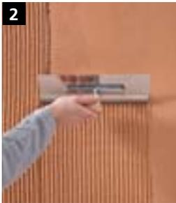
2 Apply and texture StoLevel Calce FS (colour shade 14DC400) with the rust-free Sto-Adjustable Toothed Trowel and the Sto-Toothed Blade for adjustable toothed trowel C2 or with the Sto-Swiss Large-area Smoothing Trowel toothed 6 x 6 mm.
