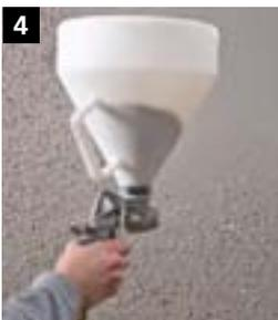
4 Immediately afterwards, use the Sto-Terrazzo Effect Gun to blow the Sto-Terrazzo Effect natural sand mixture into the wet plaster from top to bottom, using slight circular movements. Leave to dry until it feels dry when touched with the back of your hand.
