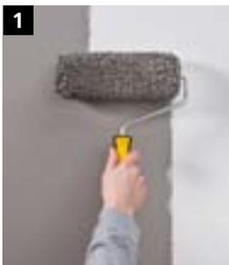
**1** Apply two coats of StoColor Opticryl Matt (colour shade 14DC170) using a short-pile roller. Leave to dry.
