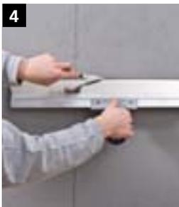
4 Create joints: place a straight edge guide (spirit level or similar) gently on the surface. Use the Sto-Plaster Molding Spatula to scrape joints into the surface, applying light pressure. Create anchoring holes: use the handle end of the Sto-Paint Roller Handle 2K to press anchoring holes into the defined points.
