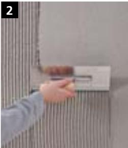
2 Apply and texture StoLevell Calce FS (colour shade 14DC350) with the rust-free Sto-Adjustable Toothed Trowel and the Sto-Toothed Blade for adjustable toothed trowel C2 or with the Sto-Swiss Large-area Smoothing Trowel toothed 6 x 6 mm.
