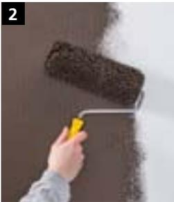
2 Simply apply the desired colour shade of StoLook Texture F (colour shade 14DC140) in a cross-wise motion using a short-pile roller. Leave to dry.
