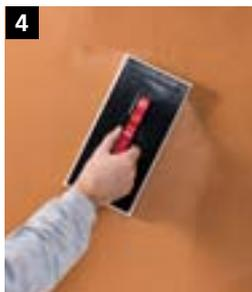
4 When the spot-smoothed finish has dried a little, use a slightly moistened (not wet) Sto-Latex Sponge to smooth it in circular movements, applying light pressure. Level ridges and tips. Smooth the surface. Leave to dry.
