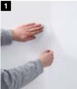
1 Evenly apply a sufficient amount of StoTex Coll to the wall in a width of 1 - 2 strips. Adapt the adhesive consistency to the mesh. Dilute with water if necessary. Insert StoTex Classic 215 S Fine without bubbles into the wet adhesive bed so that the strips abut. Leave to dry.
