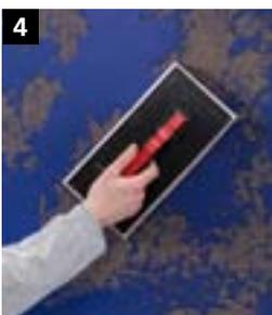
4 Smooth the individual spots and transitions to a pore-free finish using a slightly moistened (not wet) Sto-Latex Sponge on a Sto-Velcro Float Handle. Leave to dry. The final effect of the spotted coating primarily depends on the selected colour shade of StoDecolit MP.
