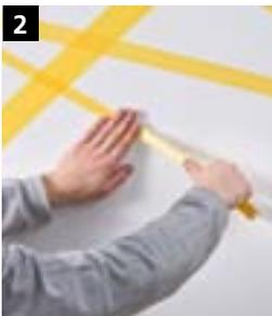
**2** Mark out the strips or areas and then mask them (3M Scotch 244 Super painter's covering tape, gold). Hint: number the masked strips according to the masking sequence.
