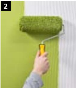
**2** Apply the desired colour shade (colour shade 14DC230) of StoColor Opticryl Gloss to the dried wallpaper using a short-pile roller. Leave to dry.
