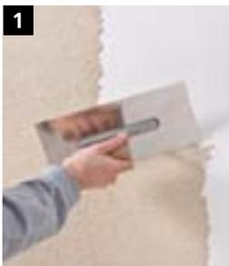
1 Use the Sto-Smoothing Trowel or the Sto-Swiss Large-area Smoothing Trowel to apply StoLevell Calce FS (colour shade natural) to grain size as a filler base coat or levelling filler coating. Smooth the surface.
