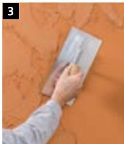
3 Apply individual patches of StoDecolit MP. Smooth the patches into irregular spots using a Sto-Smoothing Trowel held very flat, without using the edge.
