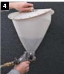
4 Use the Sto-Hopper Gun (4 mm nozzle) and an air pressure of 0.5 to blow the Sto-Silicon Carbide F54 effect mixture into the wet paint, working from top to bottom with slight circular movements. Leave to dry.
