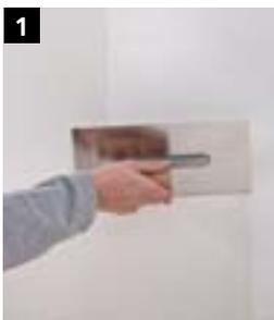
1 Use the Sto-Smoothing Trowel or alternatively the Sto-Swiss Large-area Smoothing Trowel to apply StoCalce Fondo (colour shade white) to grain size as a filler base coat or levelling filler coating. Smooth the surface.
