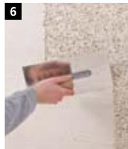
6 Spread the desired colour shade of StoCalce Active MP (colour shade 14DC190) using the Sto-Smoothing Trowel or the Sto-Swiss Large-area Smoothing Trowel so that it lightly covers the pressed-in sand mixture. Leave to dry until touch-dry.
