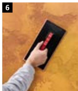
6 Dilute the second StoColor Metallic colour shade (14DC10M) to approx. 50 % with water. Apply the material thinly using a glazing spotting technique. Apply Metallic spots, spaced 50 cm apart, with the Sto-Rubber Float Sponge coarse and then immediately spread these across the entire surface. Coat the elevations with the Metallic glaze over the full surface, leaving edges and recesses unglazed.
