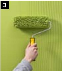
**3** Apply another coat of StoColor Opticryl Gloss using a short-pile roller. Leave to dry.
