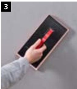
3 When the first filler and levelling coat is touch-dry, apply the second layer to grain size. Partially texture the surface with the Sto-Rubber Float Sponge coarse.
