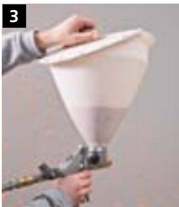
**3** Spray StoLook Texture G onto the surface from top to bottom at a distance of approx. 1.5 - 2.0 m, using slight circular movements to create an open sprinkling.
