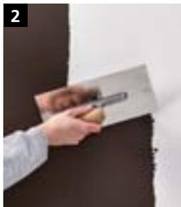
Apply StoCalce Fondo (colour shade 14DC140) to grain size using a Sto-Smoothing Trowel. Float-finish the surface using the Sto-Latex Sponge on a Sto-Velcro Float Handle. Leave to dry until touch-dry.
