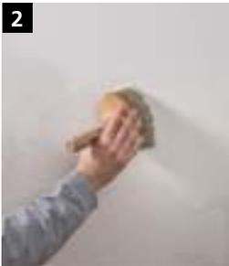
**2** Add 30 % StoLook Ballotini to StoColor Metallic (colour shade 14DC15M). Use the Sto-Wide Flat Brush Orel® mix to brush the material onto the surface in cross-wise motions. Leave to dry.
