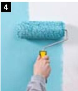
**4** Apply StoPrep In (colour shade 14DC330) to the unmasked surface using a short-pile roller. Leave to dry.
