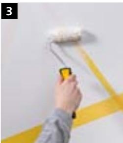
**3** To prevent the subsequent coating materials from seeping under the tape, apply StoColor Opticryl Gloss (colour shade white) to the edges of the masking tape.
