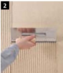
2 Apply and texture StoLevell Calce FS (colour shade 14DC190) with the rust-free Sto-Adjustable Toothed Trowel and the Sto-Toothed Blade for adjustable toothed trowel C2 or with the Sto-Swiss Large-area Smoothing Trowel toothed 6 x 6 mm.
