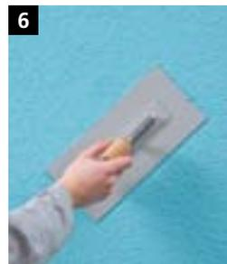
**6** Use the Sto-Plastic Smoothing Trowel to float the material using figure-eight movements.
