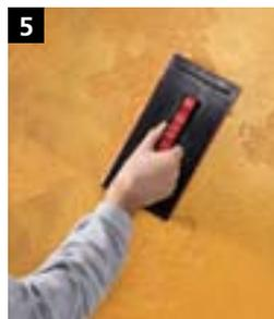
5 Dilute StoColor Metallic (colour shade 14DC38M) to approx. 15 % with water. Apply the material evenly using a short-pile roller and level out using the Sto-Rubber Float Sponge coarse.
