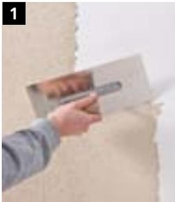
1 Use the StoCalce Marmorino Smoothing Trowel or the Sto-Swiss Large-area Smoothing Trowel to apply StoLevel Calce FS (colour shade natural) to grain size as a filler base coat or levelling filler coating. Smooth the surface.
